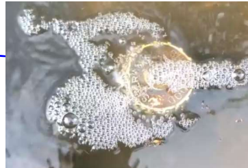
Upper O-Ring leak on underground tank
